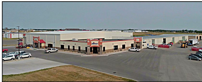
Main Office/Hardware/Service Center/Machinery Sales & Parts - Minot, ND
